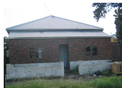
Donated house to be demolished
