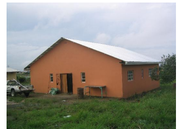
Preschool construction status on April 11, 2005
